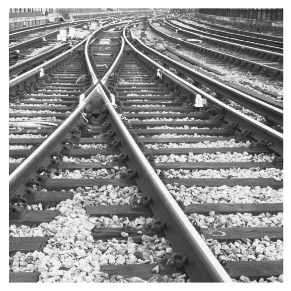
BECAUSE STEEL HAS A RELATIVELY HIGH COEFFICIENT OF THERMAL EXPANSION, STANDARD RAILROAD TRACKS ARE CONSTRUCTED SO THAT THEY CAN SAFELY EXPAND ON A HOT DAY WITHOUT DERAILING THE TRAINS TRAVELING OVER THEM. (Milepost 92 1/2/Corbis. Reproduced by permission.)
