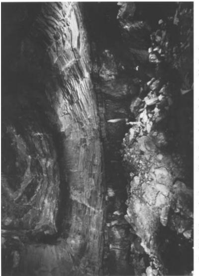
Fig. 26.4 Underground cavity created by the Gnome fusion explosion, part of the Plowshare program
