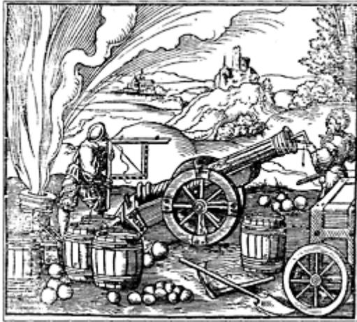
*The gunners are using a sighting device and a quadrant to gauge the proper elevation for the cannon. From Johannes Stöffler, Der...mathematischen und mechanischen Künst (1541).*
