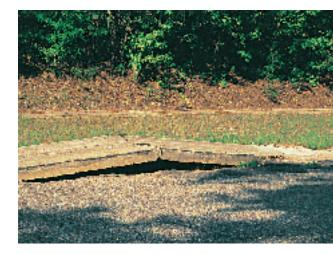
**Figure 2** Most objects expand as their temperatures increase. Pieces of this concrete sidewalk forced each other upward when the concrete expanded on a hot day.
