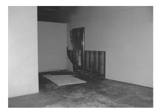
**Figure 9.16** Vapor explosion blast damage.
